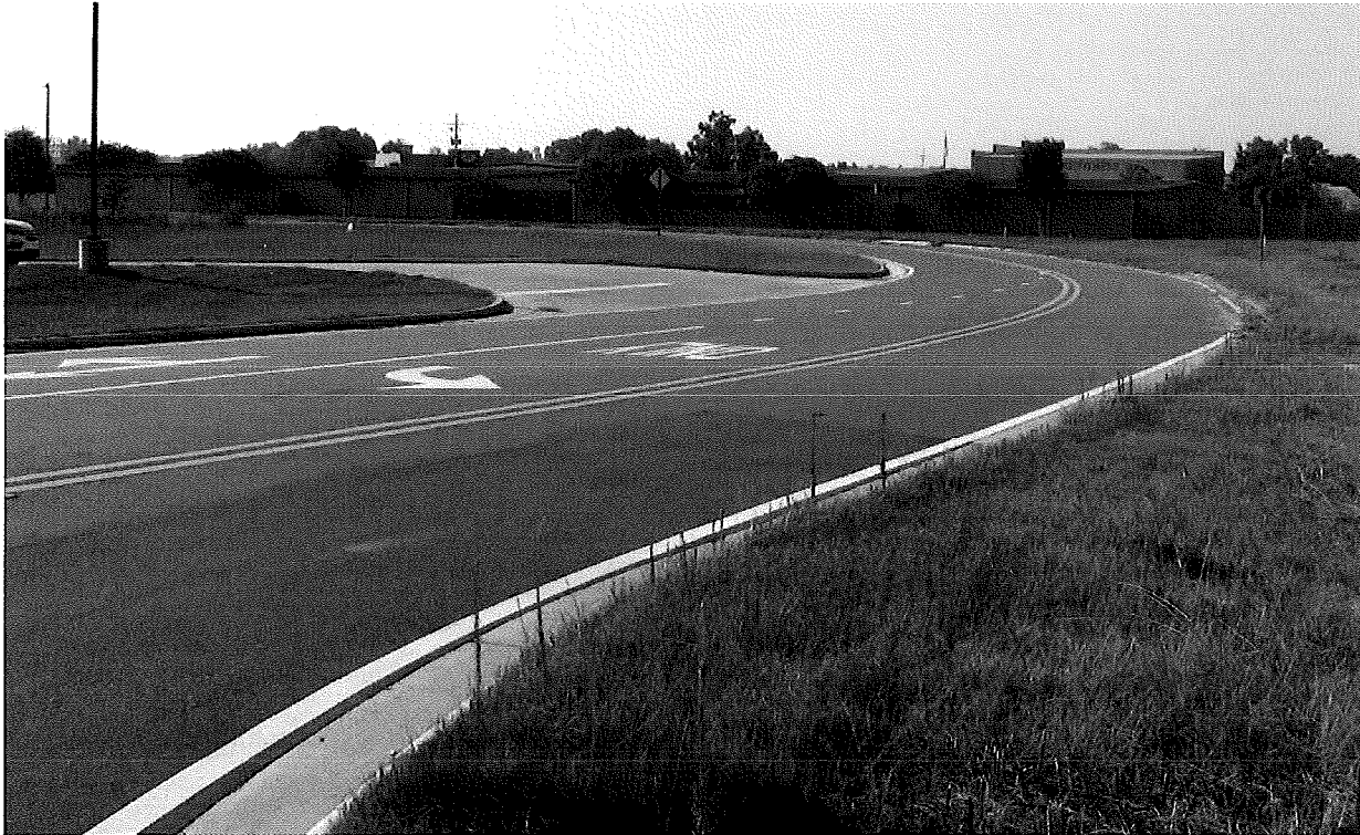
Dees Drive – Looking south from Gluckstadt Road
